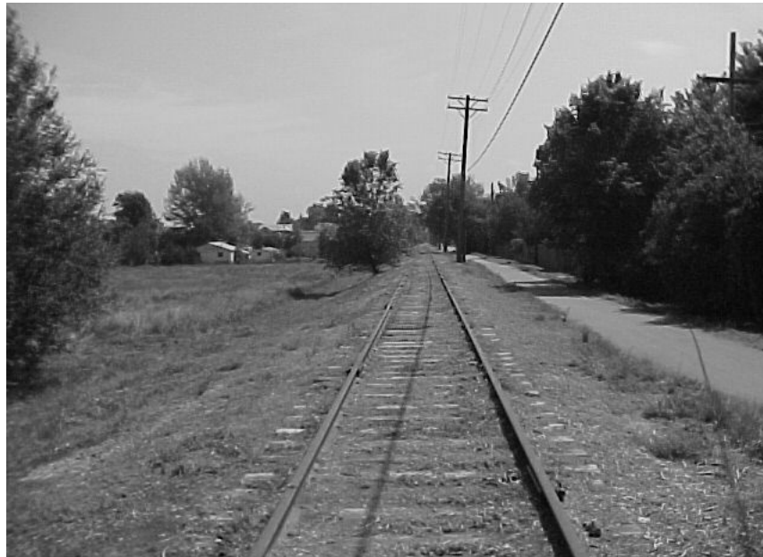
Abandoned track along 13 th Avenue.
